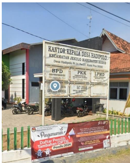
Figure 2. Hadipolo village hall (source: personal documentation)
